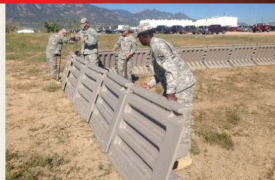
47 lb. walls are easy to handle. No special equipment is necessary for assembly.
